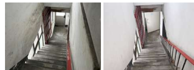
Note: Dormitory Environment Optimization Item - Painting of Stairway and Emergency Stairway Walls, Before-and-After Comparison.
