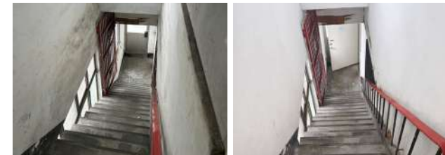
Note: Dormitory Environment Optimization Item - Painting of Stairway and Emergency Stairway Walls, Before-and-After Comparison.
